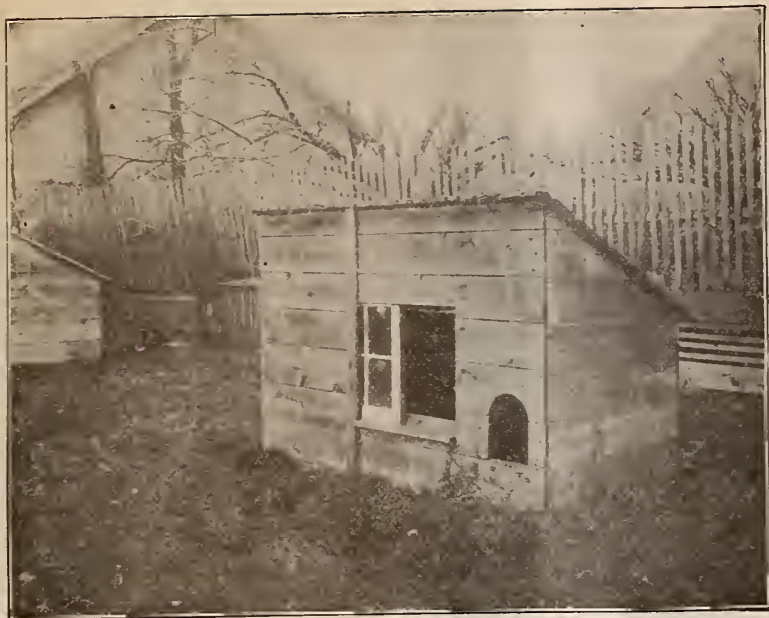
SUMMER ROOSTING COOP. Used by C. S. Mattison, So. Shaftsbury, Vt.
